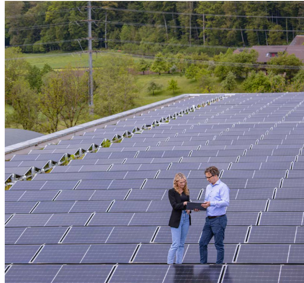
The rooftops of our Bystronic headquarters in Switzerland are equipped with photovoltaic systems that significantly contribute to powering our production operations.
